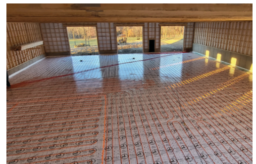
Radiant Heating is an energy efficient, quiet, allergy-friendly solution to home heating.
